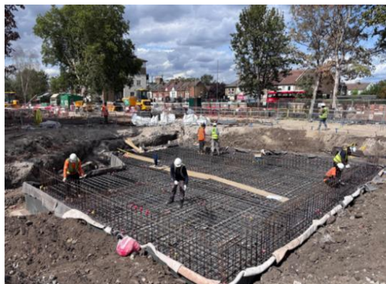
Photo (above): Block C core progressing
