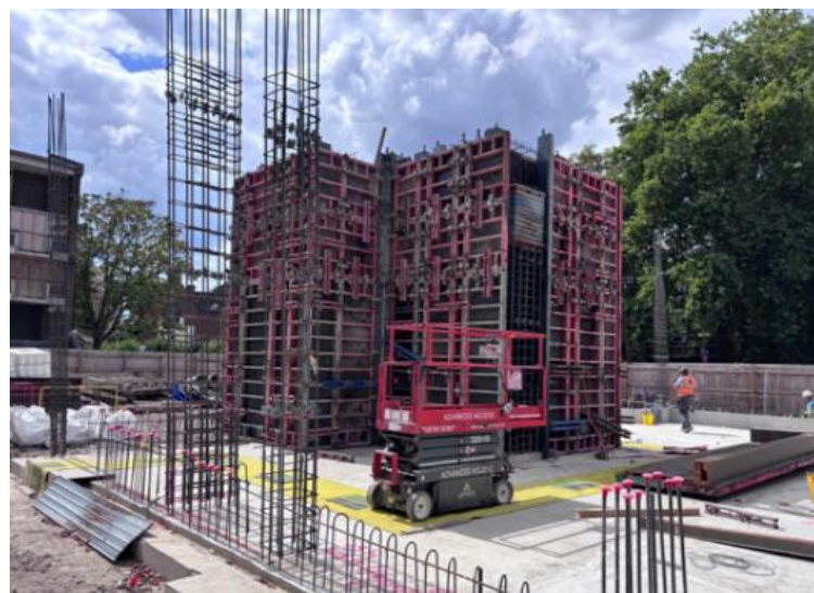
Photo (above): Block C core walls being progressed
